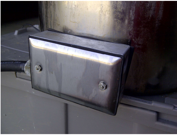
Figure 3: J-box extender with inside metal cover punched for heating element
